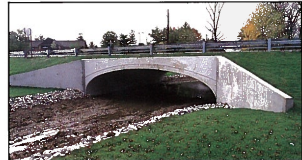
9 Finished Bridge – It is economical, durable, quickly installed and looks great.
