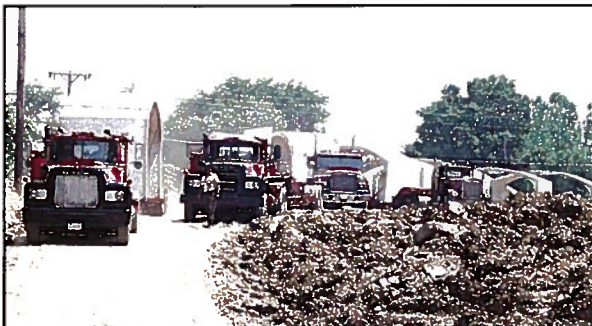
4 Transportation – Entire structure arrives on schedule ready for installation.
