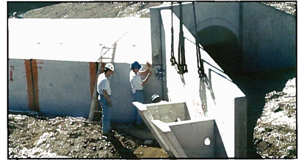
7 Wingwalls & Headwalls – Setting of precast wingwalls and headwalls completes the bridge.
